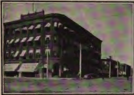
TYPICAL OFFICE BUILDING, PHOENIX
